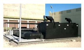
followed by MBR filtration. Two trains of treatment capacity 8,500 m³/day each constitute the plant process of which only one train currently in functional. Each train is equipped with blowers, capable of supplying airflow up to 6,000 m³/h. Odor causes nuisance to the adjacent hotel building, where hotel guests getting disturbed due to bad smells that spread over one kilometer surrounding areas, therefore odor nuisance issue needed to be solved immediately.
